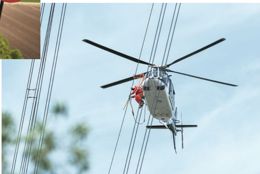
Using a helicopter to help install bird protection measures: the black-and-white markers help the birds better see the conductors.
