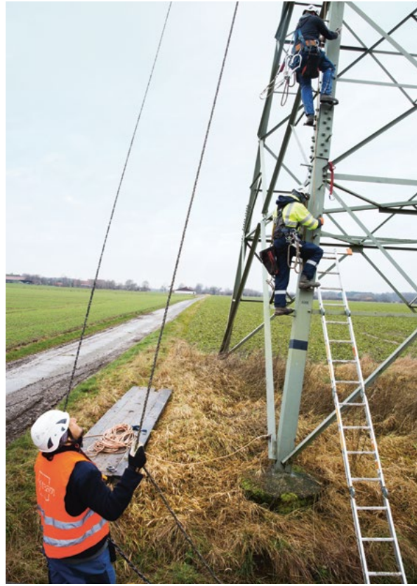
Up we go! A nesting aid is secured to Amprion pylon 133.
