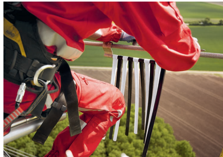
The black and white bird protection markers are mounted on the ground wire with the help of a helicopter. The poorly visible wire is thus better recognisable for birds.
