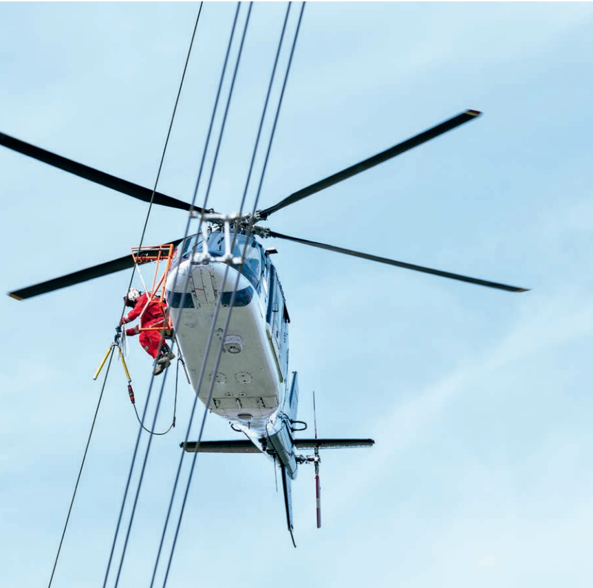
The black and white bird protection markers are mounted on the ground wire with the help of a helicopter. The poorly visible wire is thus better recognisable for birds.
